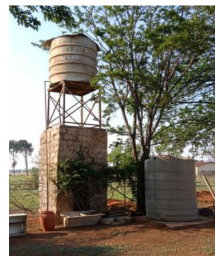
Pipes installed & new tank
